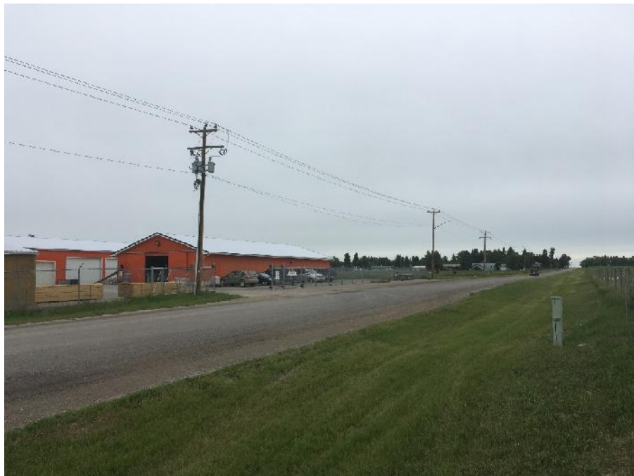
Photograph 12 – Adjacent West Road Facing Northwest Note the pole mounted transformer adjacent to the property and electrical box along road set-back.
