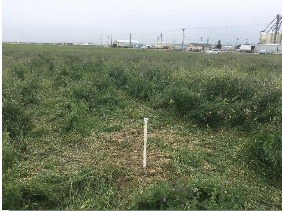
Photograph 5 – Piezometer on West Side of the Property Facing Southwest Note the piezometer was installed days before for a geotechnical investigation related to developing the Property.
