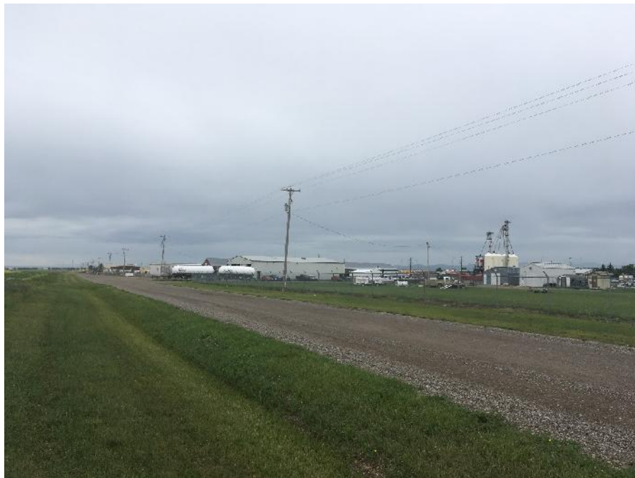
Photograph 8 – Adjacent West Properties Facing Southwest Note the pole mounted transformers along the road.
