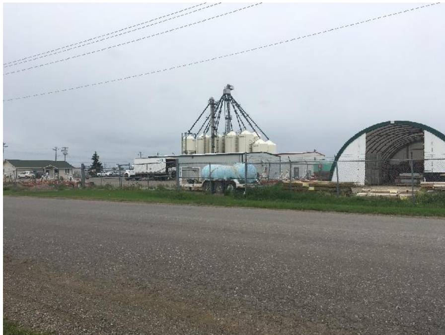
Photograph 10 – Adjacent West Properties Facing Southwest
